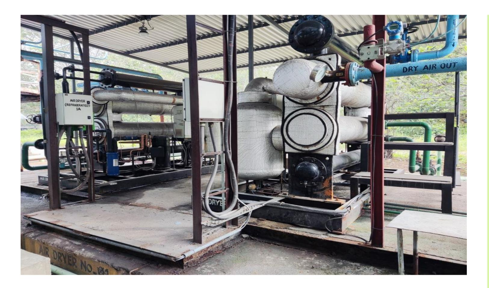
Innovation 2: 100 % Replacement of desiccant driers with energy efficient refrigerant driers
